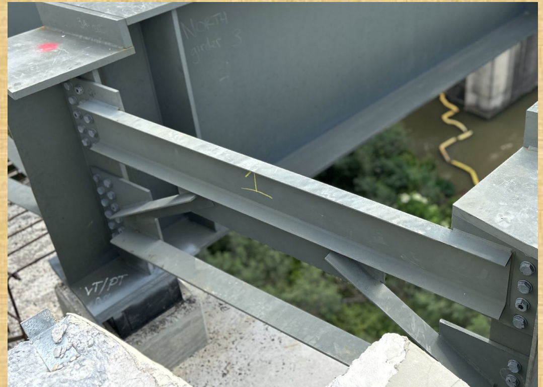
LA 23 over Intercoastal Waterway (Belle Chasse, LA)
