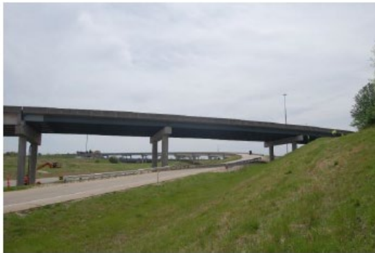
(c) large vertical clearance over a roadway
