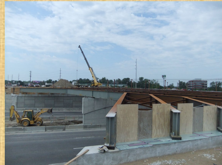
Allisonville Road over I-465 (Indianapolis, IN)
