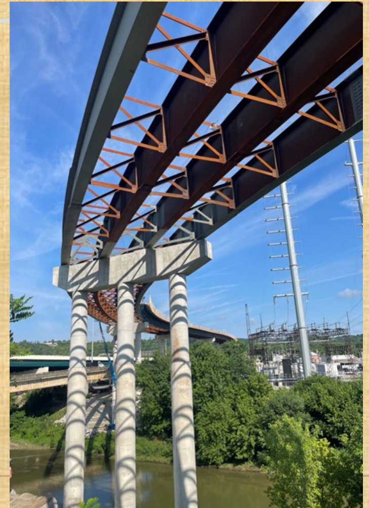
Mill Creek Expressway (Cincinnati)
