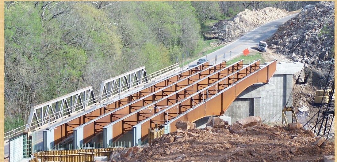
Haunched Plate Girder Bridge
