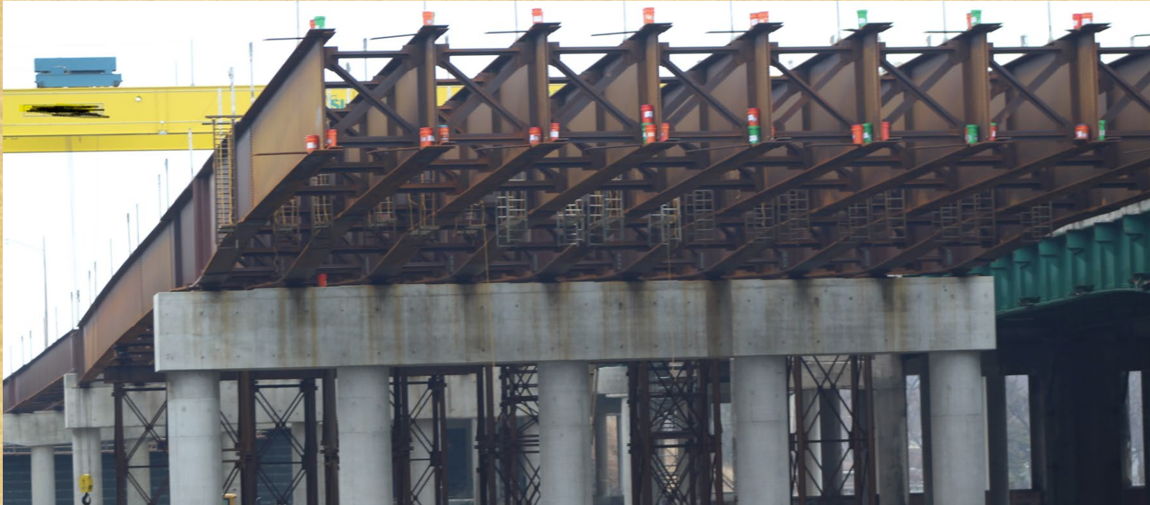
I-294 SB “Mile Long Bridge” in Chicago, IL
