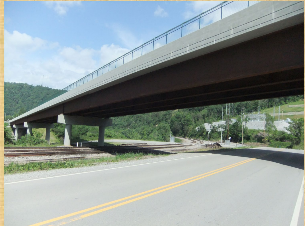
KY-80 over Russell Fork, CSX RR & Roadway
