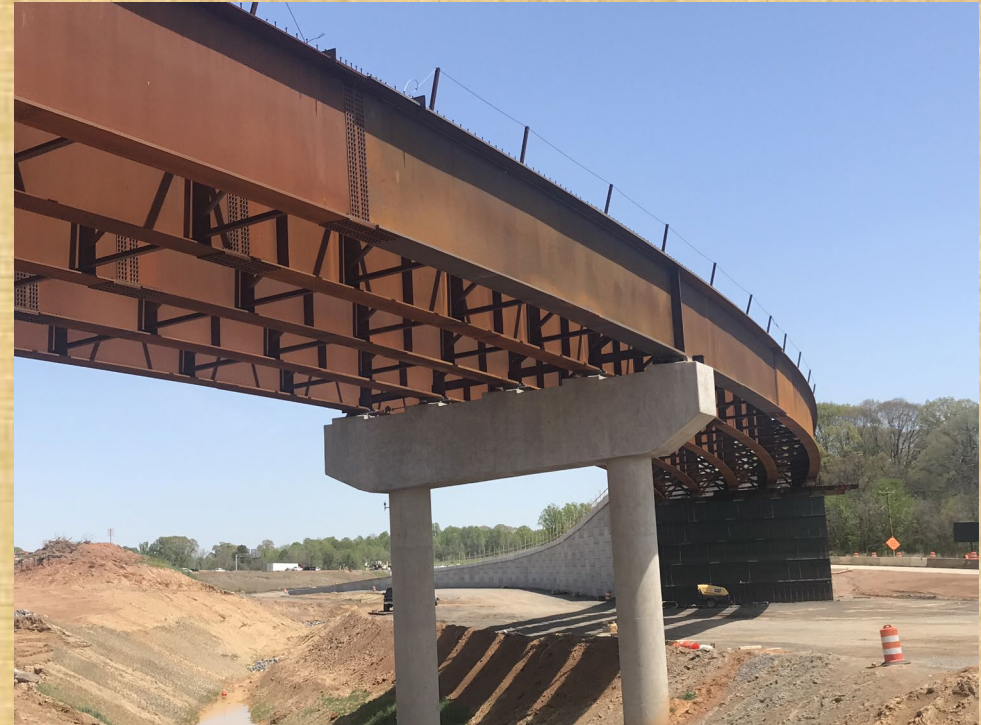
I-40/I-77 Interchange near Statesville, NC
